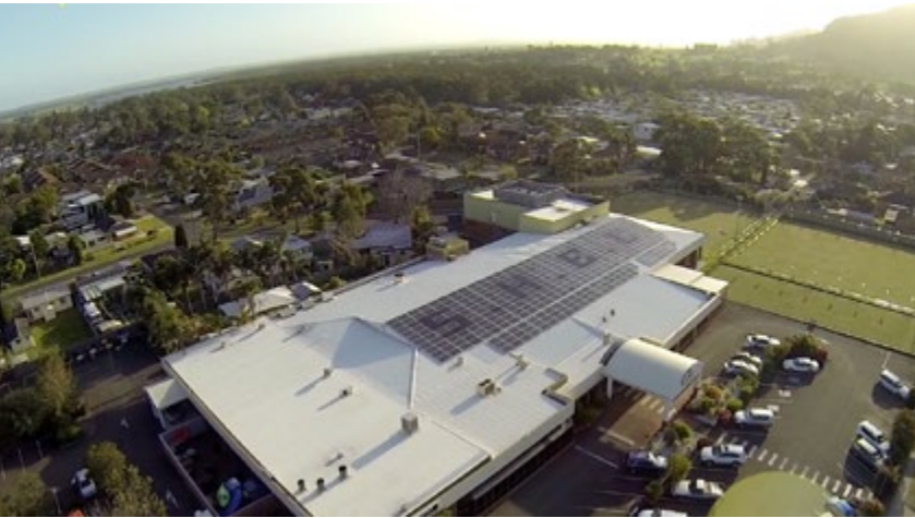
Repower One, Australia's first community investor-owned solar power system at Shoalhaven Heads Bowling and Recreation Club. 99kW, operating since August 2014. Photos courtesy of Embark.
